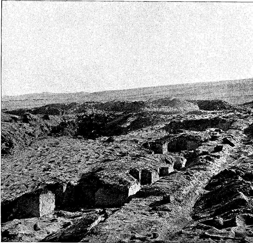
PANELLED BRICKWORK, WEST SIDE, LOOKING S.
